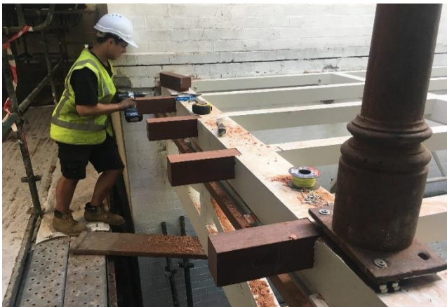
Jacob from Carfax repairing the first floor verandah frame.
